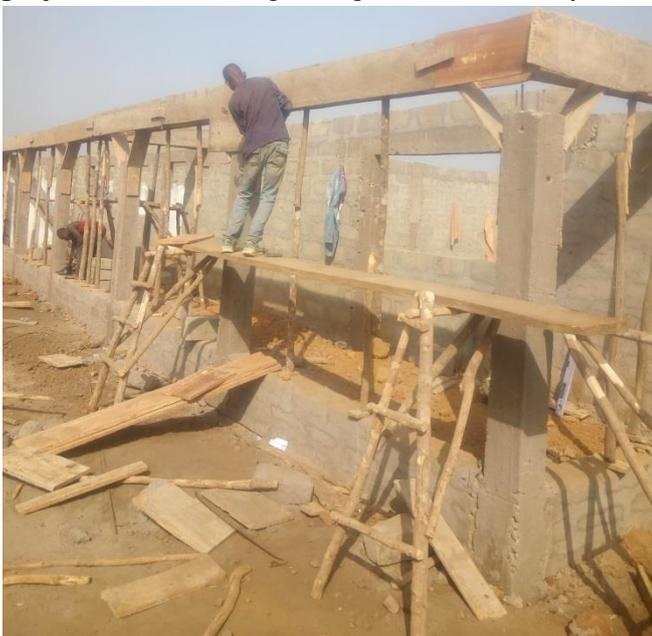
A high quality scaffold platform – it may not meet UK Health & Safety standards but it does the job ! As you can see from the next 3 photos the roof timbers were installed, the galvanised sheeting is on & this week they completed the ceilings. They have started to lay the concrete floors and when completed they will start the rendering
