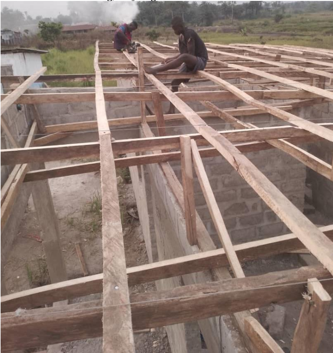
The progress is amazing – this photo was taken on Friday afternoon
